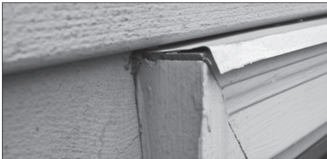
Figure 3. All too often, aluminum drip caps develop a negative slope. The usual consequences include corner dribbling and casing rot. [Photo credit: Jeff May, author of The Mold Survival Guide from Johns Hopkins University Press.]
