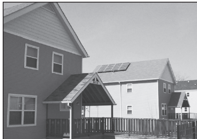
Figure 1. Twelve of the houses at the New Homes for South Chicago III development are equipped with roof-mounted photovoltaic arrays. In most of these houses, the furnace uses far more electricity than is produced by the PV systems.
